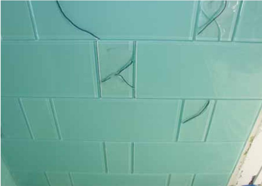
ANSI product and installation standards recommend a mortar setting bed thickness of  $\frac{3}{32}$  to  $\frac{1}{4}$  inch (nominal) and recommend against using thinset to flatten a substrate. This is especially important when setting glass tile, as an excessively thick setting bed will shrink as it dries, which can cause tiles to crack, particularly when the shrinkage is uneven due to variations in mortar application thickness (differential shrinkage).
