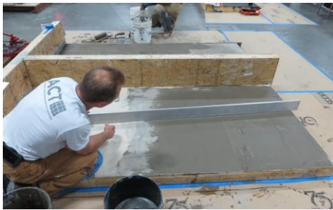
Substrate Prep being completed for LFT and SP Test
