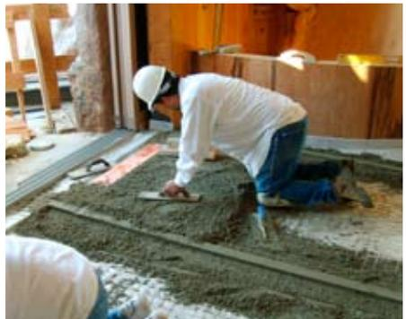
*Like natural stone, a thick set mortar bed can be used when installing large format tile.*
