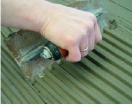
*A medium-bed (thin-set) method, utilizing large trowel sizes and mortar with anti-slump characteristics, is most common when installing large format tile.*
