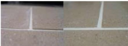
*Large format tile set in a staggered pattern can exacerbate lippage that is more obvious with narrow grout joints.*
