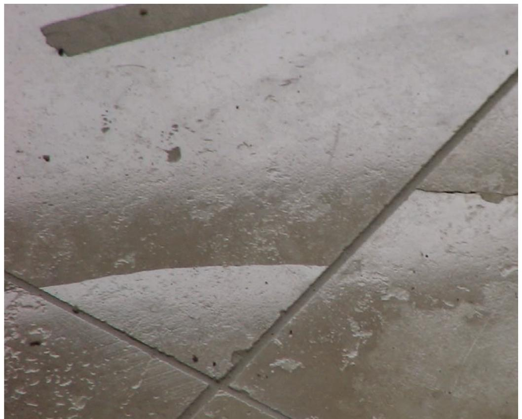
**Right: “Poor mortar coverage can result in unsupported hollow spots that make tile susceptible to cracking from concentrated weight.” Photo courtesy Ceramic Tile and Stone Consultants.**
