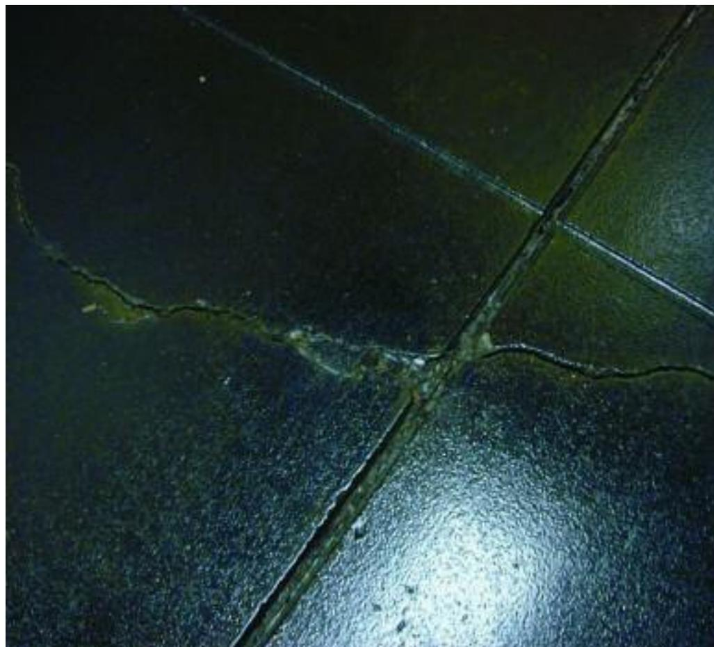
**Right: Cracked tile may be due to shrinkage of a concrete subfloor or deflection in a wood subfloor.**
