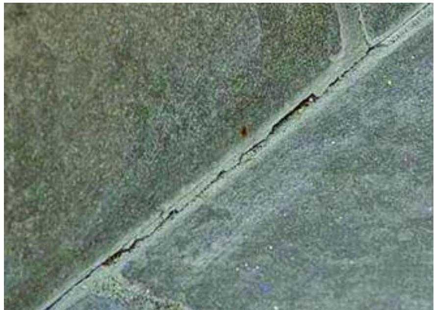
**Right: Grout cracked at wall/floor transition due to substrate movement; use movement joints per TCA EJ-71.**
