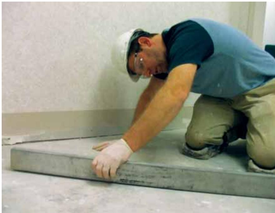
For thin-bed installations, installers check for variations in concrete with a straightedge. Although a slab may meet the flatness tolerances called out in the concrete portion of the specification, it may not be flat enough for a ceramic tile installation, particularly if large tiles are chosen.
