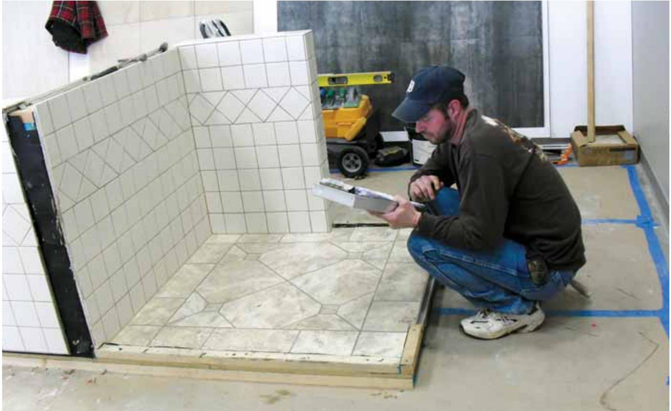
*Ceramic Tile Education Foundation evaluators carefully inspect test modules to determine if the installer will be certified.*
